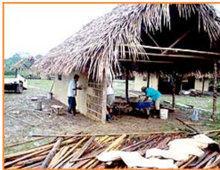
Two tribal villages are being built near Punta Gorda
